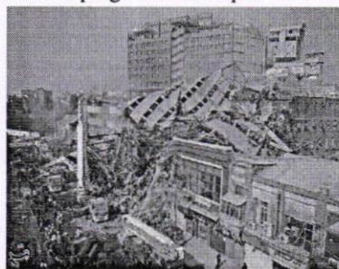
Fig 2 Plasco Building Progressive Collapse
